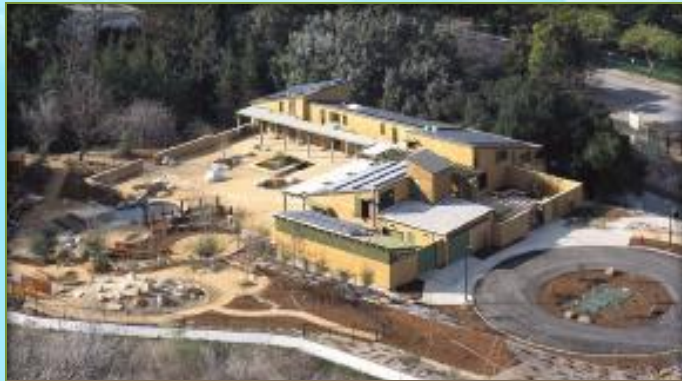
The Audubon Center at Debs Park LOS ANGELES, CALIFORNIA
